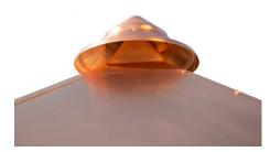
the lid of a box) over the top of the turret. The border on its lower edge is bent outwards to prevent rainwater from trickling over the surface of the turret (drip-stopping effect).
